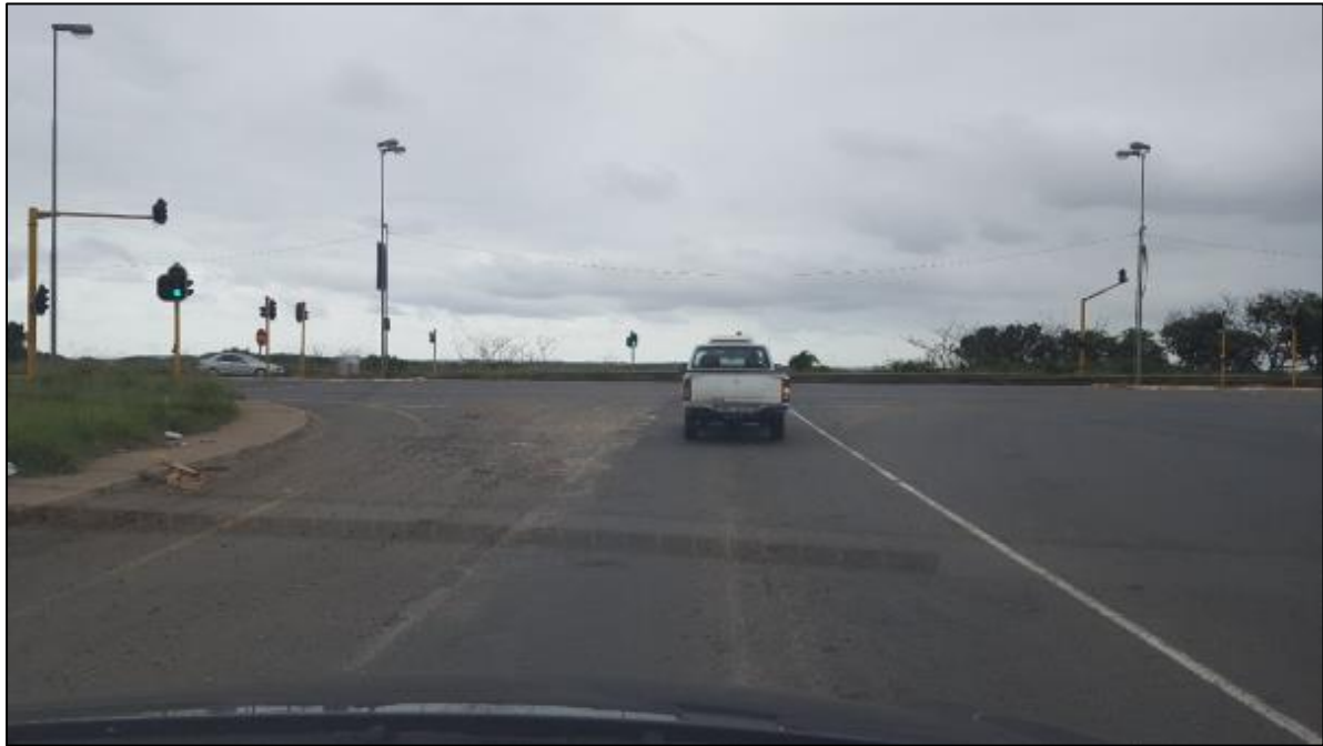
Picture 4 – Western Arterial signalised junction with the John Ross Highway
